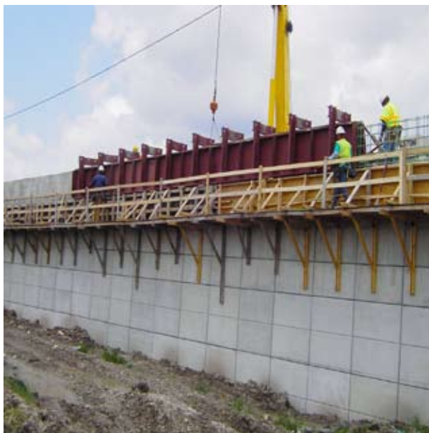
BELOW: CAST-IN-PLACE BARRIER IS BEING POURED ON TOP OF THE T-WALL® UNITS.
