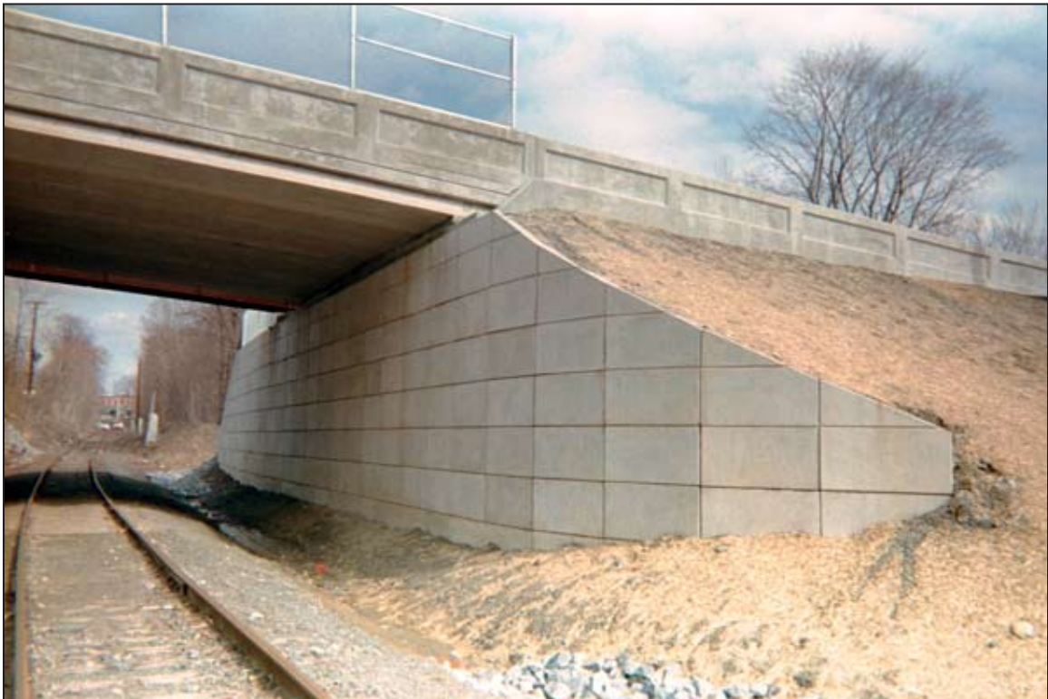
Finished abutment with wrap around wingwall –
